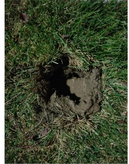
Downspout pop-ups that are covered over with dirt, roots, or grass needs to be cleaned and exposed to ensure proper function.
